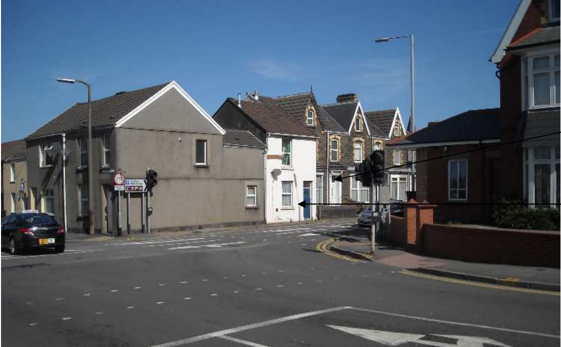
Figure 3 – View across junction to Victoria Gardens
